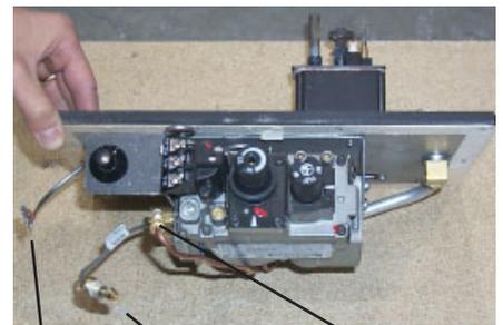
Thermopile Wire Thermocouple Wire Pilot Nut
