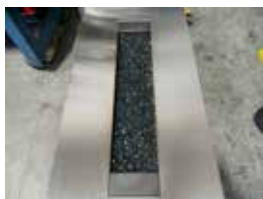
3. Work Crystals downwards to front edge of top edge of burner.
