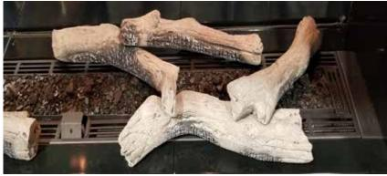
15. Install Log 8 between Log 3 and Log 4, as shown below.
