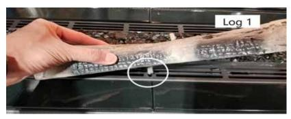
7. Lay the log on the firebox. Ensure the bottom left end of the log is 3/4" away from the edge of the firebox.
