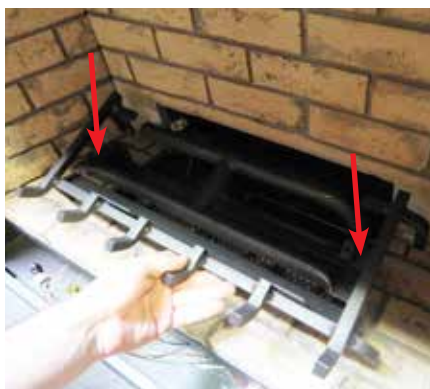
Diagram 1: Remove left and right screws.
