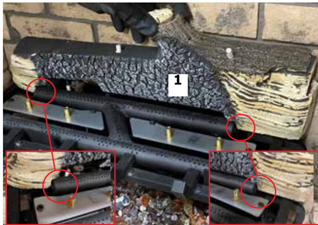
Diagram 6-Log 1 installation
