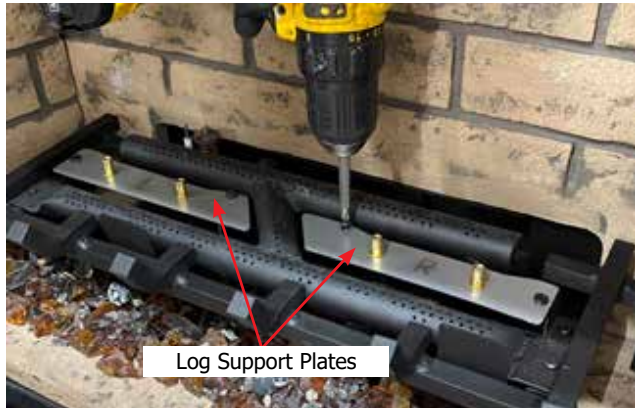
Diagram 5-Install Log support plate installation
