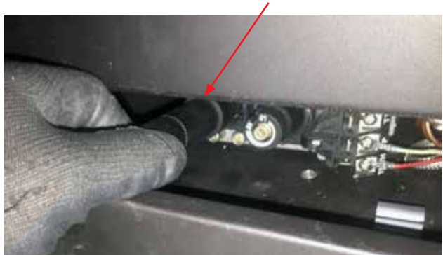
Extender knob slid over on/off/pilot knob on gas valve
