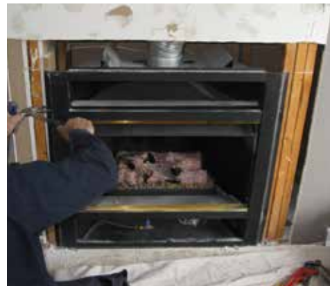
Remove unit from framing
