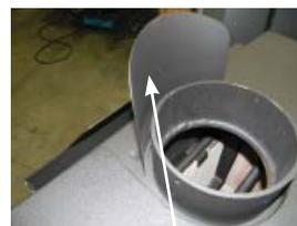
Installed Pipe Shield
