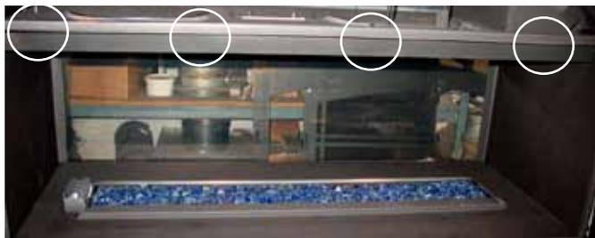
3) Loosen screw securing the panel clip located in the middle of the side panel - inside the firebox.
