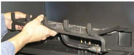
Schéma 1: Remove the left and right screws and then lift out the burner/grate assembly.
