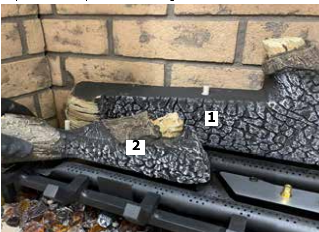
Diagram 7-Install Log 2
