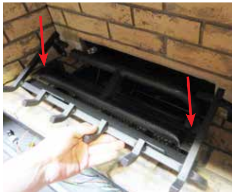
Diagram 1: Remove the left and right screws.
