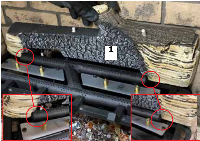
Diagram 6-Log 1 installation
