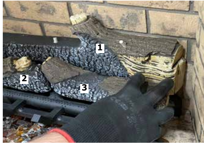
Diagram 8-Install Log 3
