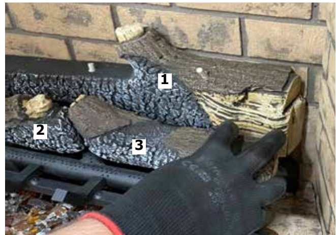
Diagram 8-Install Log 3
