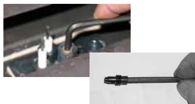
Diagram 2: Slide burner assembly to the right—then remove.
