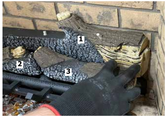
Diagram 8-Install Log 3
