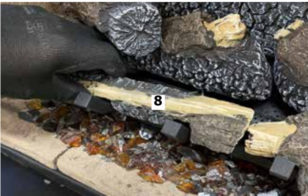
Diagram 13-Install Log 8
