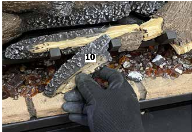
Diagram 15-Install Log 10
