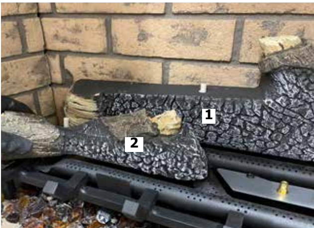
Diagram 7-Install Log 2
