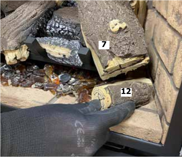
Diagram 17-Install Log 12
