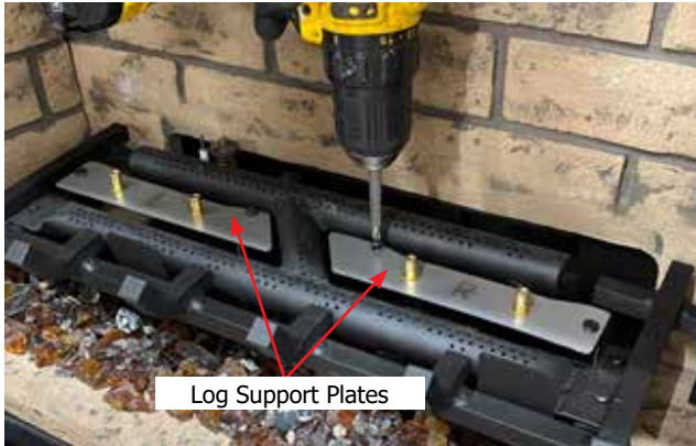
Diagram 5-Install Log support plate installation
