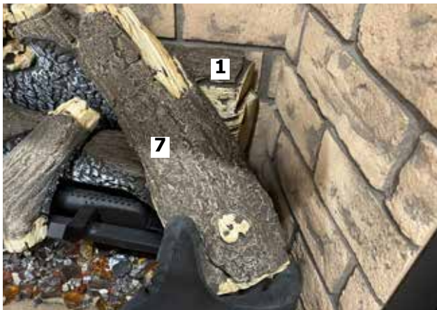
Diagram 12-Install Log 7
