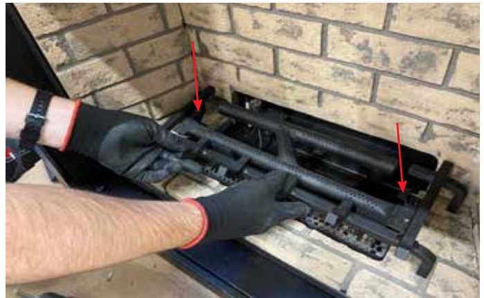
Diagram 2-Log Grate Install
