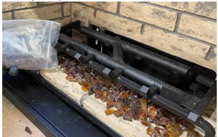
Diagram 3-Install Glass
