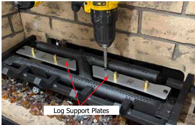
Diagram 5-Install Log support plate installation
