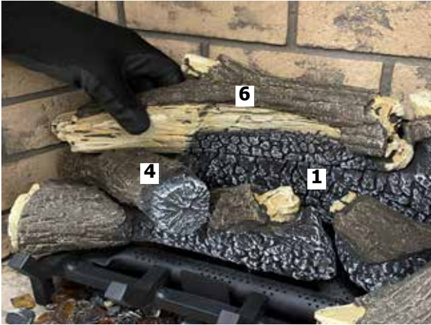
Diagram 11-Install Log 6
