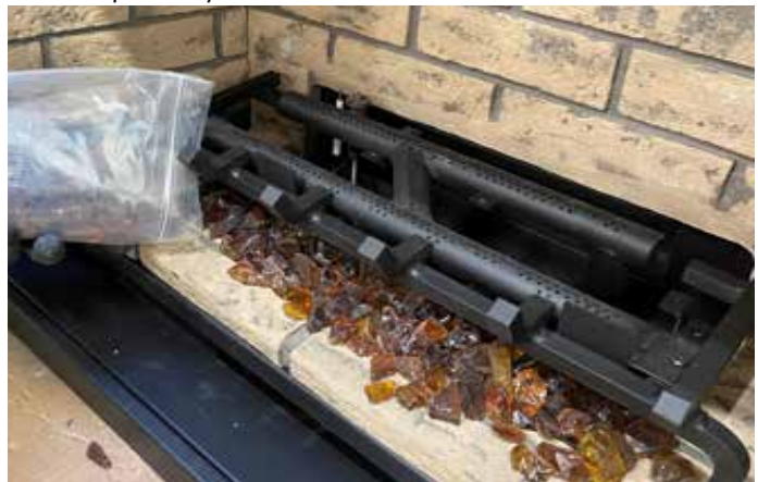
Diagram 3-Install Glass
