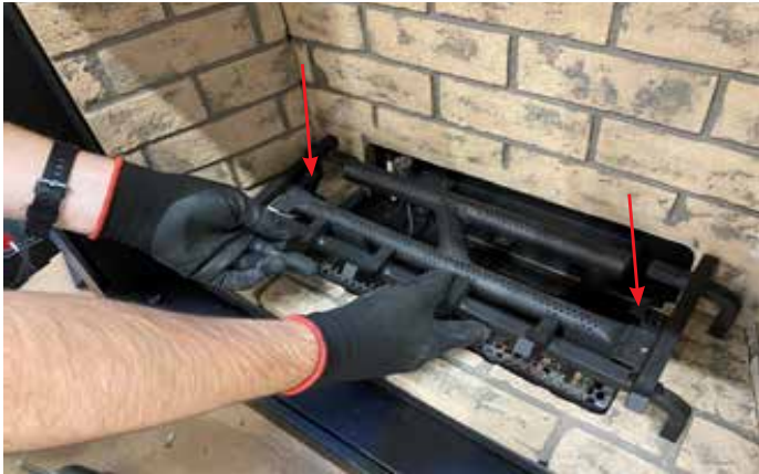
Diagram 2-Log Grate Install
