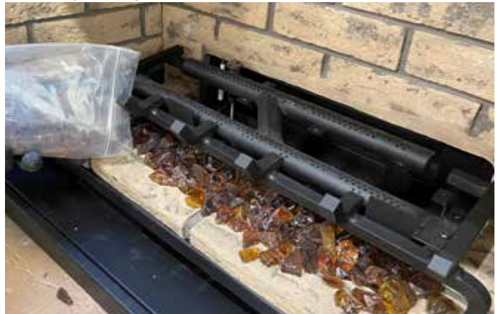
Diagram 3-Install Glass
