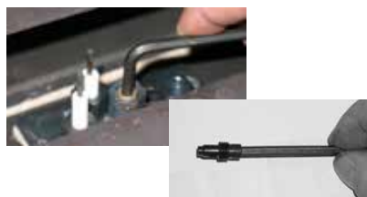
Diagram 2: Slide burner assembly to the right—then remove.
