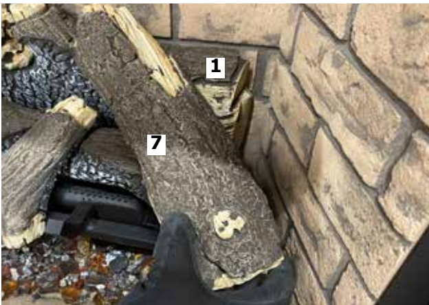
Diagram 12-Install Log 7
