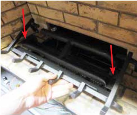
Diagram 1: Remove the left and right screws.
