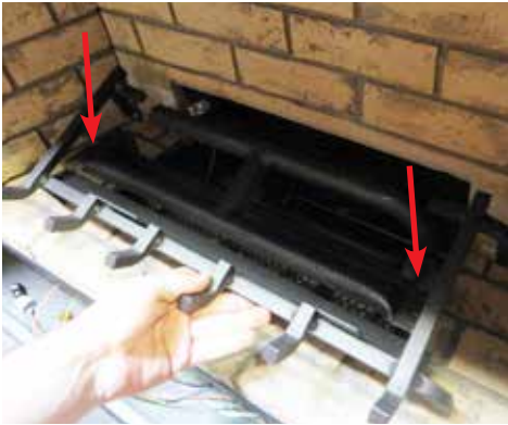
Diagram 1: Remove the left and right screws.
