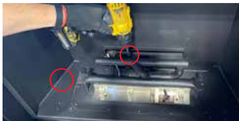
Diagram 2: Slide burner assembly to the right—then remove.
