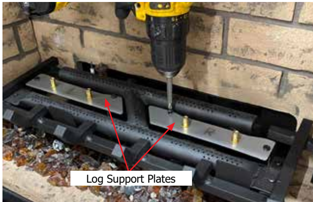
Diagram 5-Install Log support plate installation
