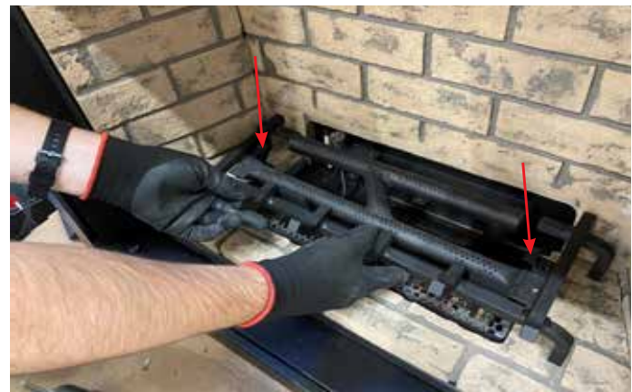
Diagram 2-Log Grate Install
