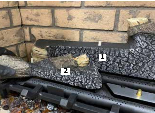
Diagram 7-Install Log 2
