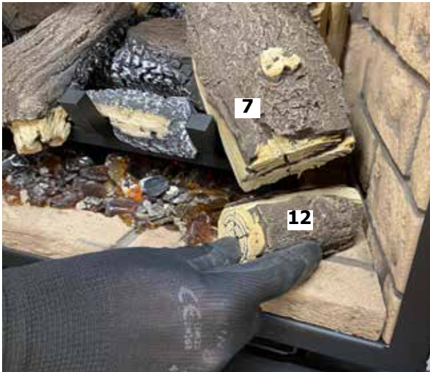
Diagram 17-Install Log 12
