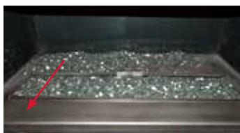
3) Work Crystals from back to front edge of Firebox Floor
