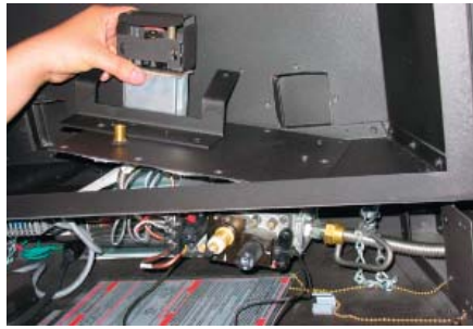
Diagram 5: Lift out Valve Tray Assembly
