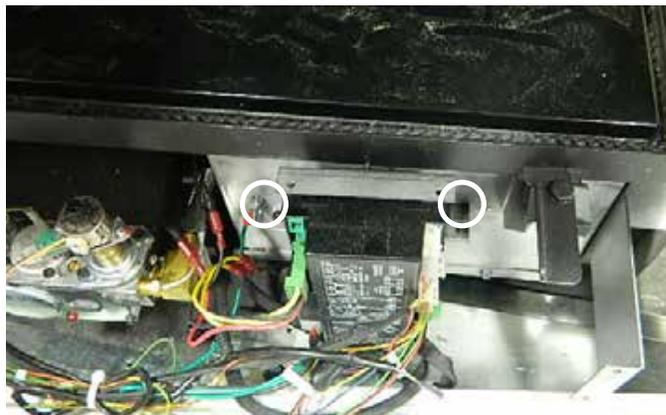
7. Remove and discard 2 Pressure regulator screws (A) using a (T20 or slot screwdriver,) Pressure Regulator (B) and Spring and Diaphragm (C) (see below).
