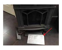
Fold down access door, and then remove two screws as shown below
