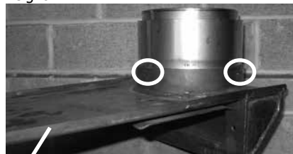
Diagram 2 Flue Adaptor
