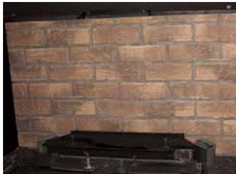
Back Panel Installed
