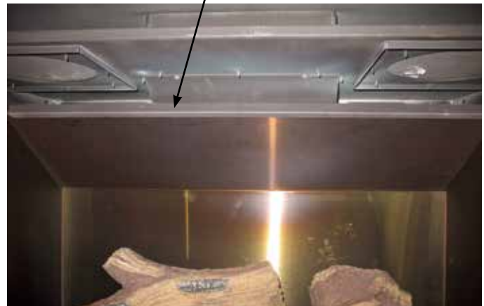
Top panel bracket shown installed with Stainless Steel Panels
