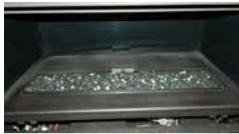
1) Start installing Crystals on the Burner (NG, Propane, ULPG)
