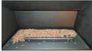
1) Start installing Crystals on back of Burner and Firebox Floor
