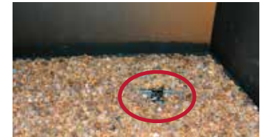
5) Ensure Crystals DO NOT block the front of the pilot hood and flame to light the burner
