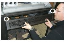
3) Attach the Bottom Louver or Grill to the hinges on the bottom flange of the fireplace.
