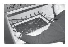
5) Remove the burner assembly by removing the 4 Phillips head screws and then slide the burner assembly away from the orifice and lift out.
