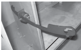
Hinge with door removed.
