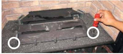
Diagram 1: Remove the left and right screws.
