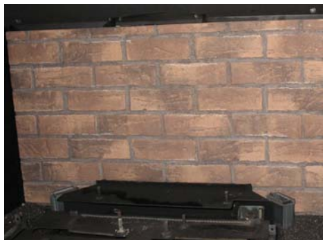
Back Panel Installed
