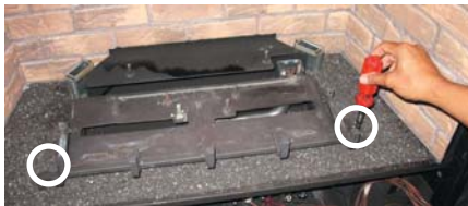
Diagram 1: Remove the left and right screws.
