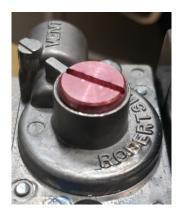
6. Apply conversion label to gas valve and install supplied vermiculite on the burner.
