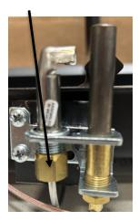
2. Unscrew nut, NG pilot orifice can now be removed.
