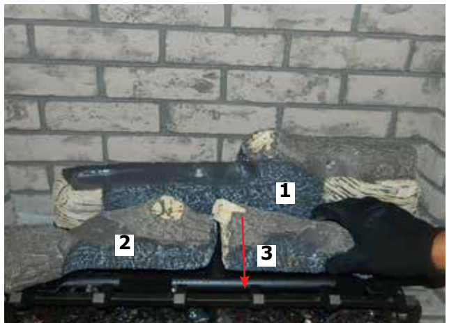
Diagram 9—Install Log 3
