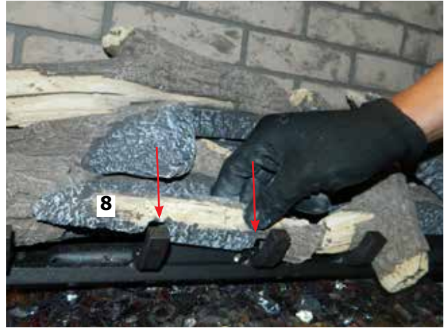
Diagram 14—Install Log 8
