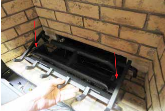
Diagram 2—Log Grate Install
