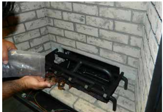
Diagram 3—Install Glass
