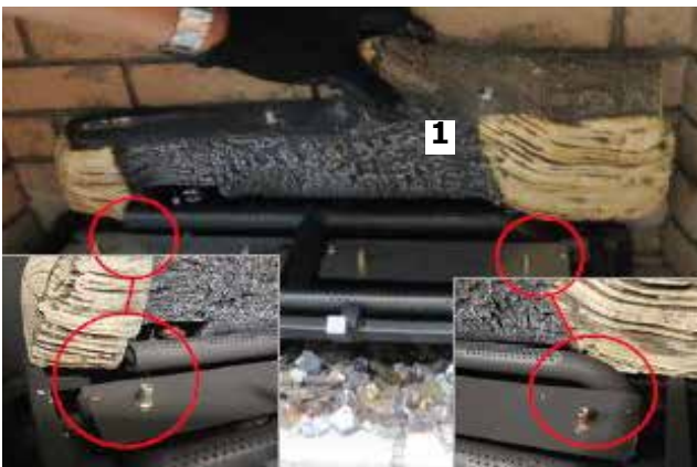
Diagram 7—Log 1 installation
