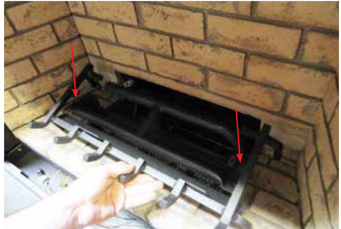
Diagram 2—Log Grate Install
