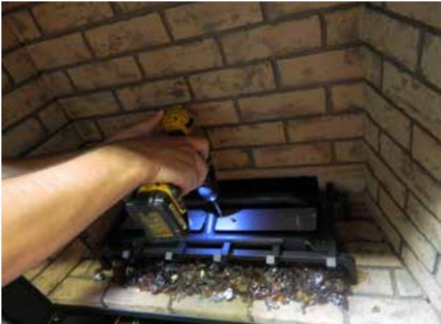
Diagram 5—Install Log support plates
