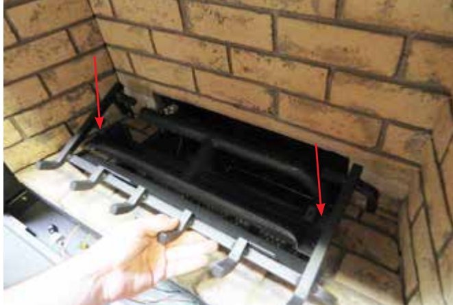
Diagram 2—Log Grate Install
