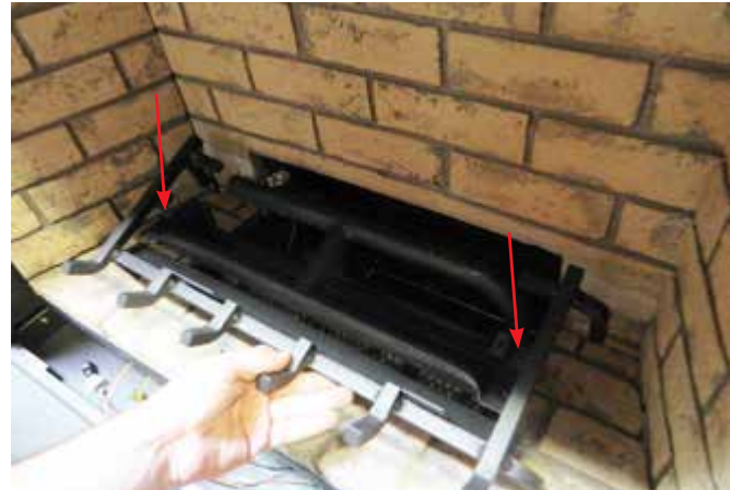
Diagram 2—Log Grate Install
