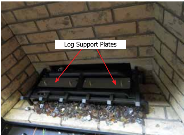
Diagram 6—Log support plates installed
