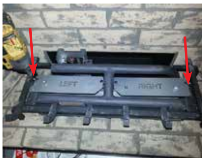
Diagram 1: Remove the left and right screws.
