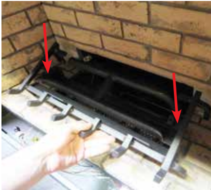
Diagram 1: Remove left and right screws.
