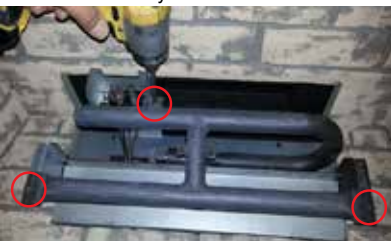
Diagram 2: Slide burner assembly to the right—then remove.
