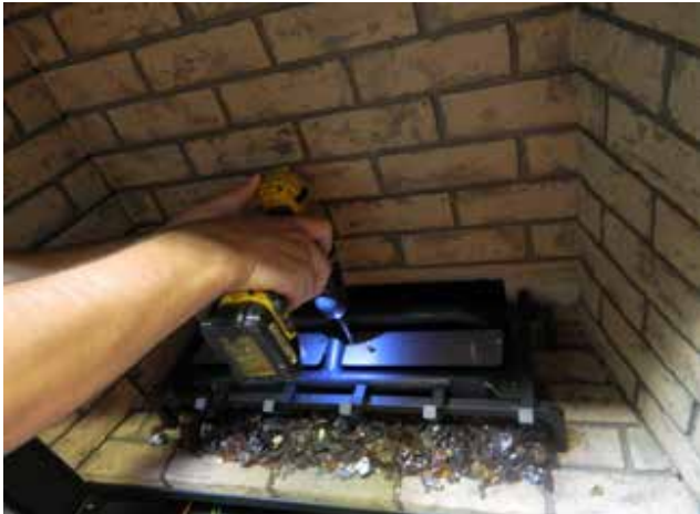
Diagram 5—Install Log support plates
