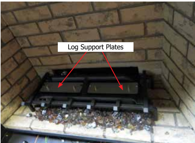
Diagram 6—Log support plates installed
