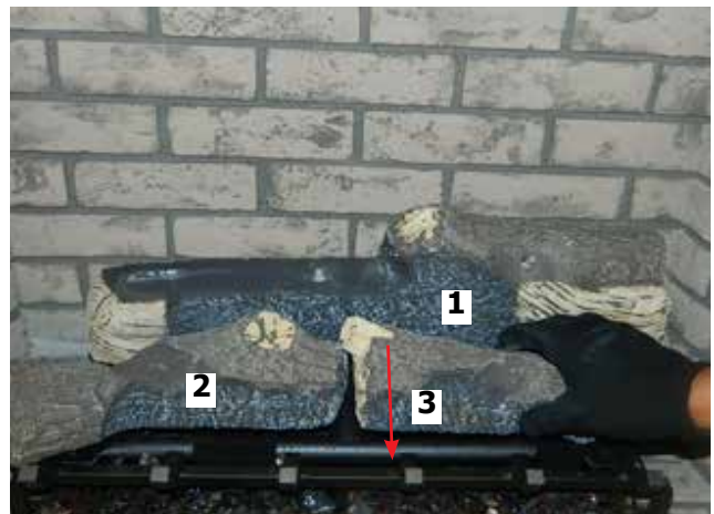
Diagram 9—Install Log 3
