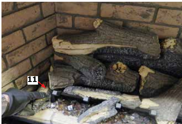
Diagram 17—Install Log 11
