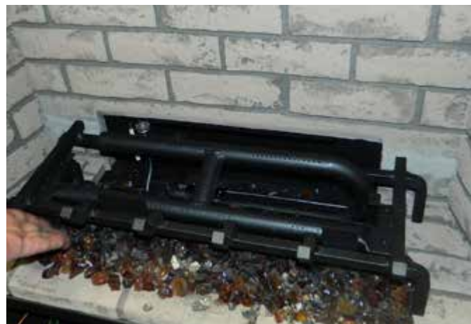
Diagram 4—Install Vermiculite + Lava
