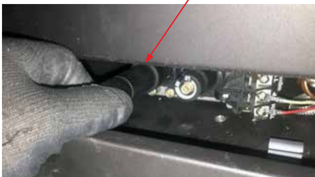
Extender knob slid over on/off/pilot knob on gas valve
