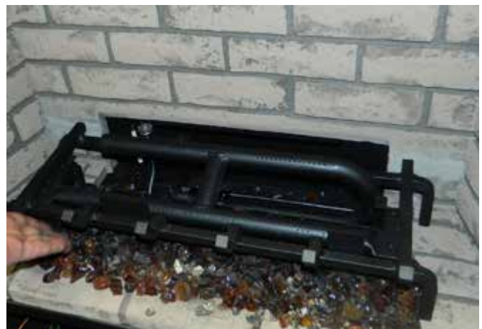
Diagram 4—Install Vermiculite + Lava
