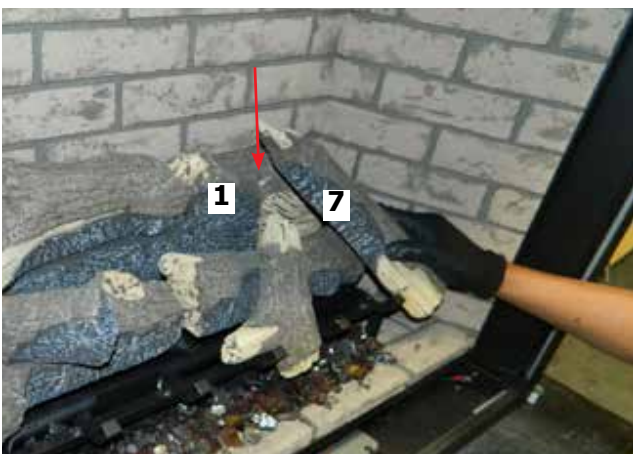
Diagram 13—Install Log 7
