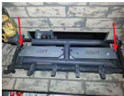
Diagram 1: Remove the left and right screws.
