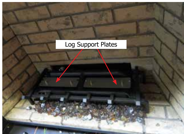
Diagram 6—Log support plates installed
