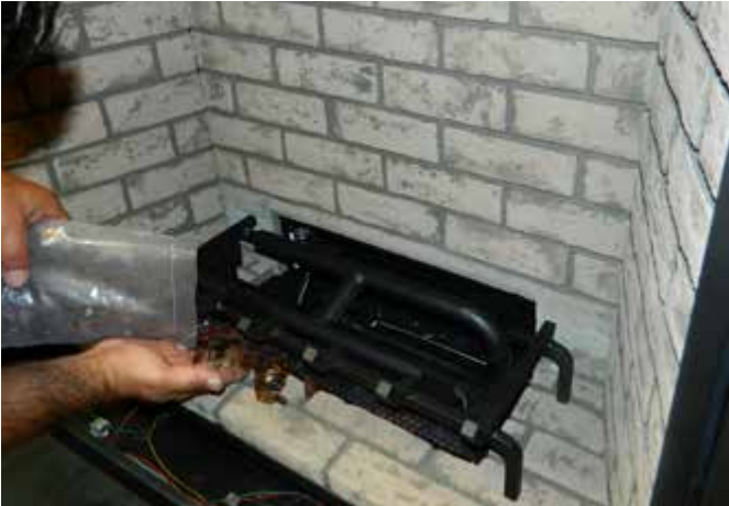
Diagram 3—Install Glass
