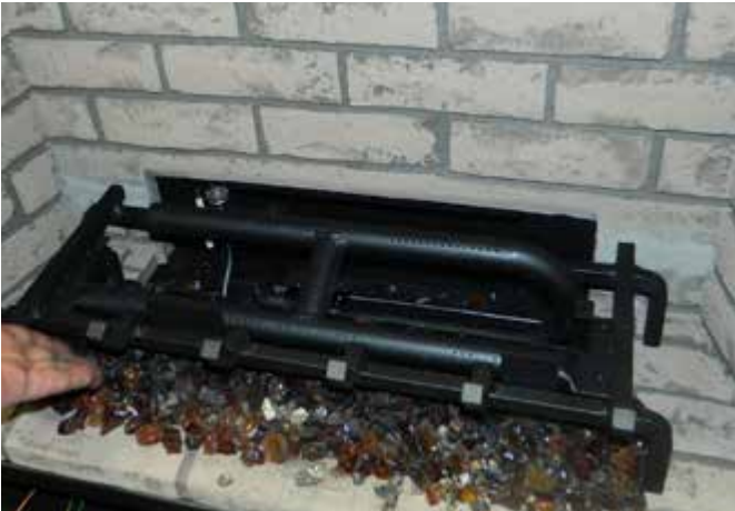
Diagram 4—Install Vermiculite + Lava
