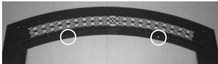
*Remove screws from the mounting tabs.*
