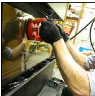
Handle glass with supplied vacuum clamps
