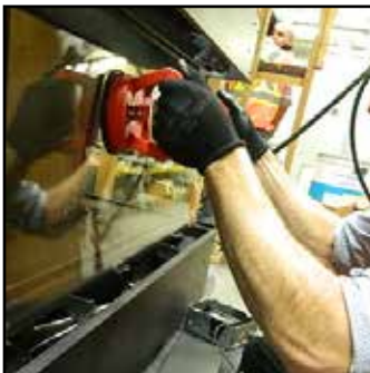
Handle glass with supplied vacuum clamps
