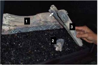
Line up pin locator and pin, Logs 1,3
