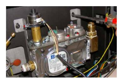
8) Remove the Gas Valve by lifting upwards and outwards.
