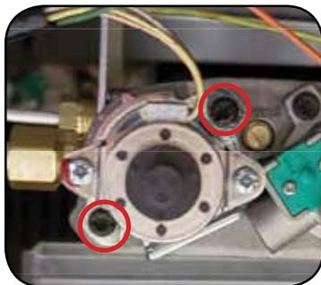
15. Connect the LP stepper motor to the receiver (same port as NG stepper removed from in Step 13), reinstall access panel.
