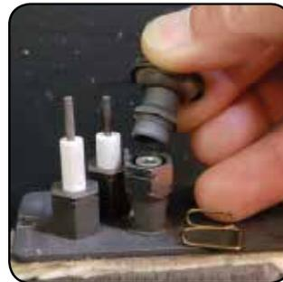
8. Unscrew the pilot orifice with the supplied Allen key and replace with the LP pilot orifice in the kit --replace pilot cap.
