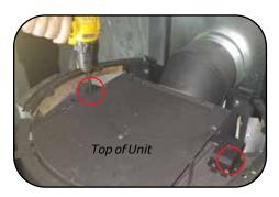
4. Remove 2 screws to release each bulb housing.
