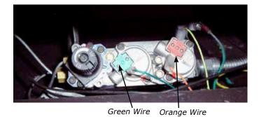
4) Disconnect the green ground wire from the valve bracket.
