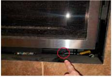
This Surefire switch is located at the bottom right center, behind the front wall.
