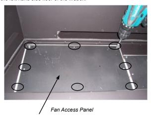
**13)** Manoeuvre the fan into position on the floor of the unit. Tilt the fan to get through the fan access panel and into position.
