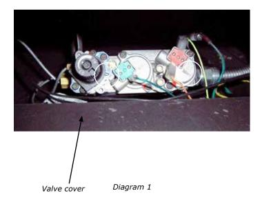
3) Slide the valve cover upward.
