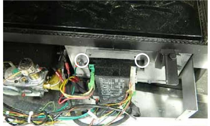
7. Remove and discard 2 Pressure regulator screws (A) using a (T20 or slot screwdriver,) Pressure Regulator (B) and Spring and Diaphragm (C) (see below).
