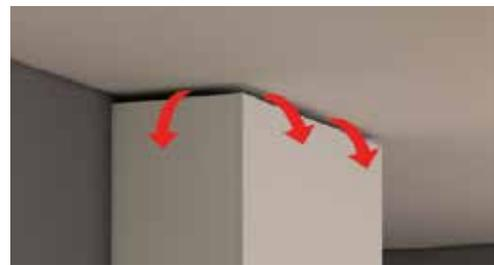
The ventilation opening may be fully open at the top of the enclosure. This type of ventilation opening would be used when the top of the enclosure is not visible from above and where the ceiling within the room is higher than normal. When creating this type of ventilation opening, measures should be in place to avoid having objects of any type falling or be thrown into the ventilation opening. Mesh screen or other preventative measures should be put into place.
