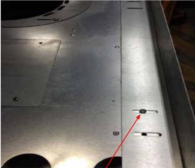
Support strip installed with slotted side on unit. The slot allows the movement of the support strip to be adjusted depending upon thickness of finish material.
