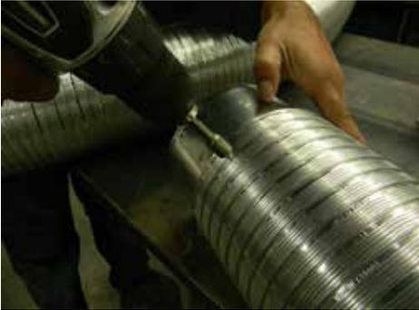
2. Attach the 4.5m duct within this kit to the connecting collar on the opposite end with the screws provided. Extend the flex to the desired length.
