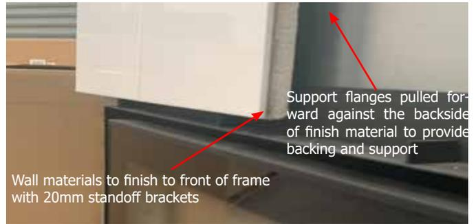
10. Install the top front wall timber frame as per minimum clearances to combustibles (page 9). Secure the top support flange to the vertical studs (left & right sides), along with the left & right support flanges.
