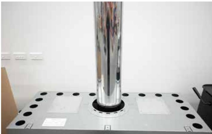
3. 8" and 10" galvanised skin fitted Air cooled bracket positions 8" inside shell and 10" outside shell – note crimped end up on outer is down.
