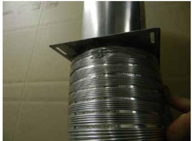
5. Cut a hole on your pre-determined outside wall to allow the fresh air hood to be installed. Install and secure the fresh air hood. Caulk around the flange to ensure tight seal against exterior of home. Join the 150 mm diameter flex from the unit adapter to the fresh air hood on the inside of the wall.
