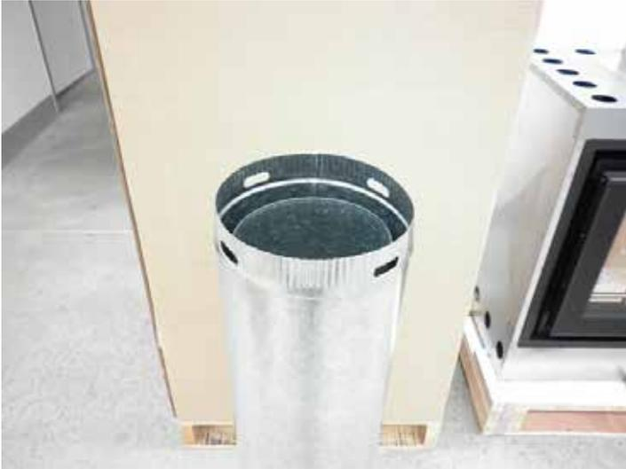
At this stage of the installation the unit is installed with the flue system and any optional kits. The next step is to install and set the support flanges in the correct position to accommodate the front wall framing and finishing.
