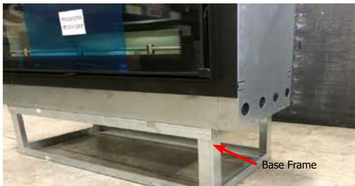
2. Position your base frame in the predetermined location of fireplace. Level then mark the position of the base frame. Remove the frame and set aside.
