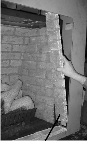
Right Side Exterior Brick Panel
