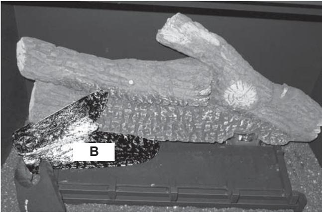
5) Place Log A on the front right side of the burner. Position the notch on the bottom right side of the log into the right side of the grate.
