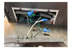
13. Tuck wires neatly into the unit using the cable ties and clip wire holder and re-install the side cover.
