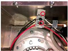
3. Ensure the replacement capacitor leads are inserted correctly into the terminal block with the red and white wires coming from the power flue harness.
