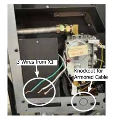
10. Add the red anti short bushings to either end of the armored cable. See below.
