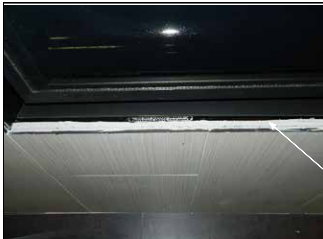
Figure 100: Top View - exposed non combustible materials
