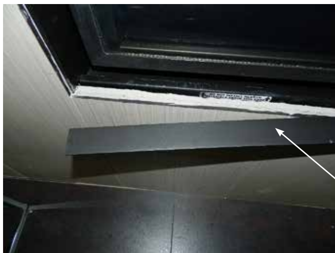
Figure 101: Top View - Sliding trim into place
