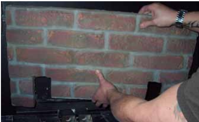
Figure 77: Lower Back Brick Panel
