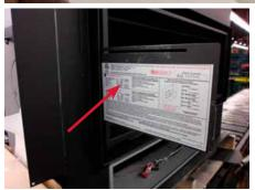
Remove Faceplate (see manual for instructions) with the faceplate removed, the rating plate will be located on the left hand side of the unit. It will be located in-between the inner and outer firebox (see picture).
