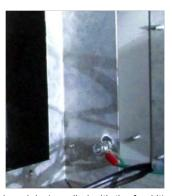
10. The fan control module (supplied with the fan kit) secures to the side access panel. Remove 2 top screws and loosen 2 bottom screws to remove the side access pane
