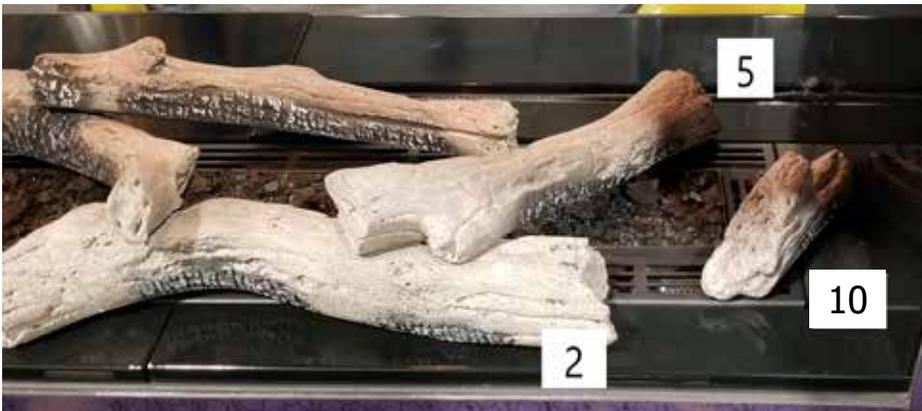
19. Install the desired optional media around the burner. You can add a maximum of 30 pieces of Andiron embers on top of the burner. **Make sure the burner surround is only 50% covered.**
