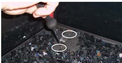
HZ33CE - install bracket, left side
