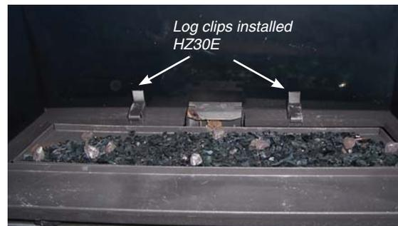
2. Position Back Log (1) by positioning centre of Log on centre of pilot hood. Rest Log 1 on log clips. Each end should rest on the lip of the burner tray – as shown below.
