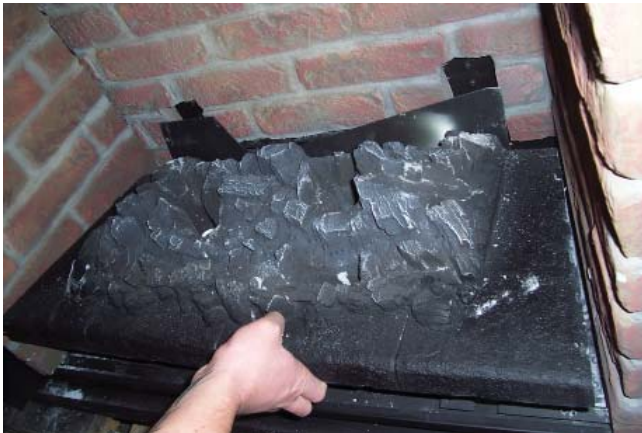
Figure 79: Burner Removal
