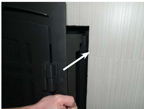
Figure 101: Line up Tabs with slot on Unit
