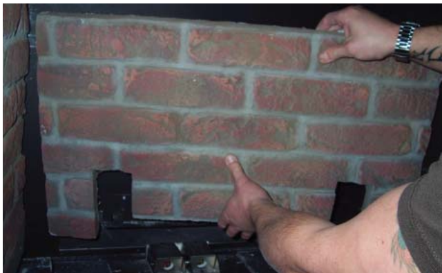
Figure 82: Lower Back Brick Panel
