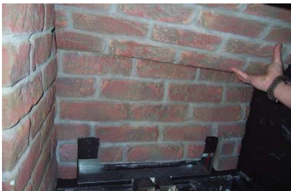
Figure 83: Upper Back Brick Panel
