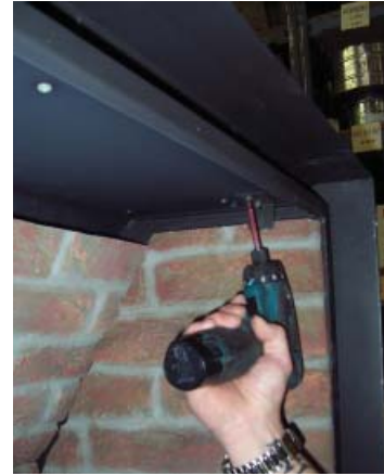
Figure 84: Right Side Brick Panel
