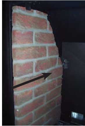
Figure 81: Left Brick Panel Install
