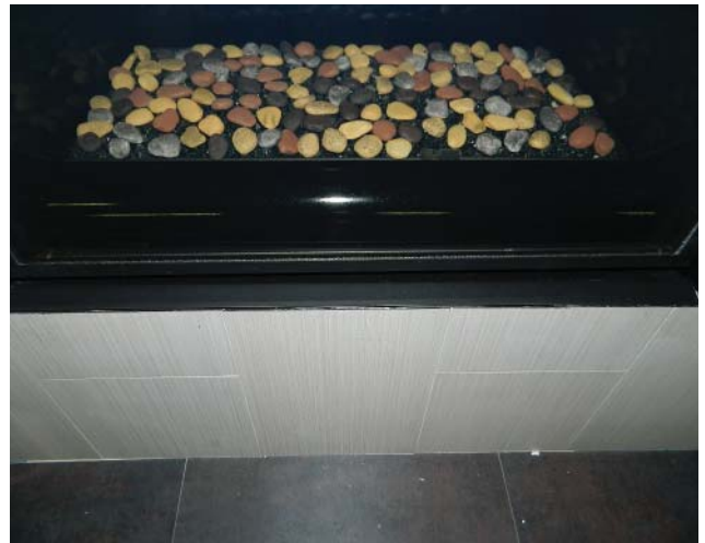
Figure 105: Completed Trim install
