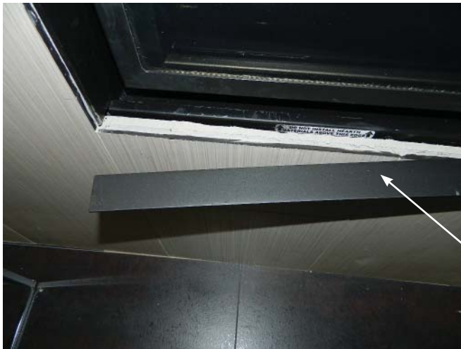
Figure 104 Top View - Trim sliding into position
