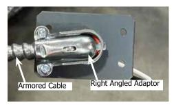
10. Install bracket onto side cover. Two holes may have to be drilled using a 1/8" bit prior to install, using the bracket as a template.
