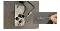
11. Remove the burner orifice with a 3/8" wrench and replace it with the #54 orifice in the kit. Use another wrench to support behind the elbow when removing/ replacing the burner orifice.
