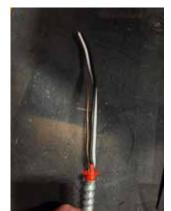
9. Install armored cable & right angled adaptor onto bracket.
