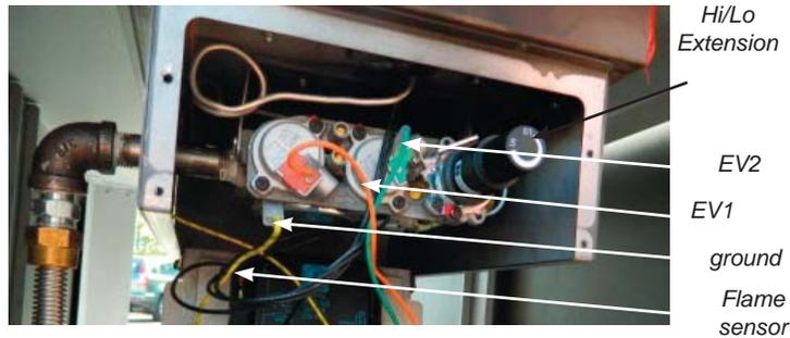
7) Remove 10 screws in locations shown below to remove valve tray.
