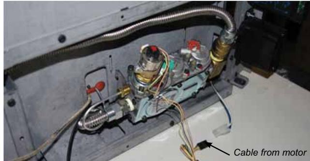
3) Disconnect the Cable coming from the Pressure Regulator Motor.
