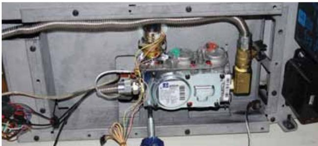
2) Loosen both screws at the top of the valve about 1/2 way out. Lift the valve body and lean outward. The Valve Brackets will rest open as shown on the right.
