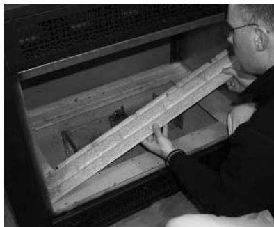
Remove the 2 Long Base Brick Panels
