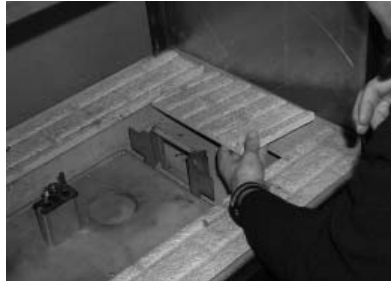
Remove Left & Right Side Base Brick Panels
