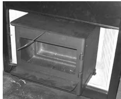
Diagram 5 Pull Rod In Place
