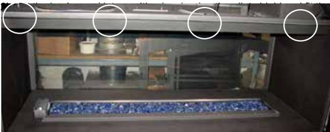
3) Loosen screw securing the panel clip located in the middle of the side panel - inside the firebox. The screw is on the top inside of the firebox.
