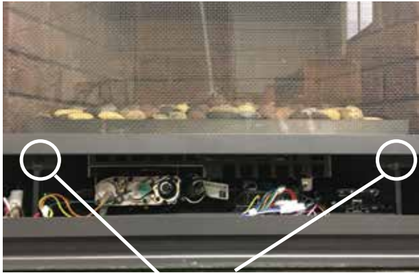
Retainer Screws Diagram 13.1
