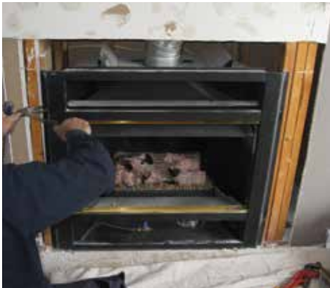
Remove unit from framing
