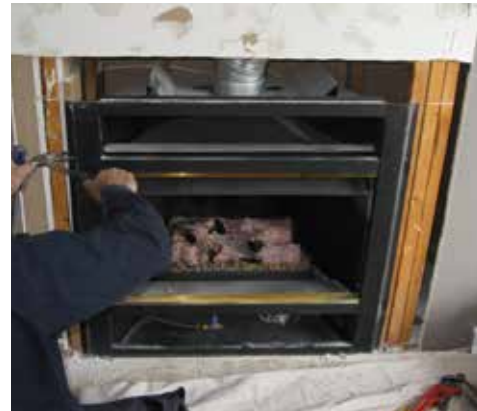
Remove unit from framing
