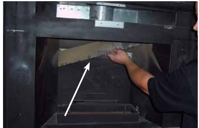
Remove rear baffle
