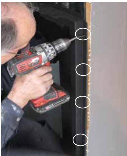
Use 4 screws on each side to secure surround to studs.
