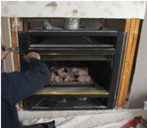
Remove unit from framing
