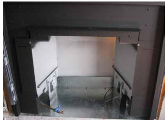
Outside firebox shown in position - refer to measurements (Step 18) before securing to surround.
