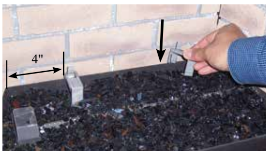
Brackets installed 4" from outside edge of burner tray
