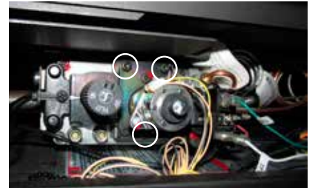
Remove NG Stepper motor and replace with LP Stepper motor
