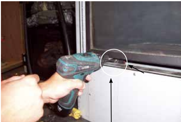
Lower mesh mounting brackets
