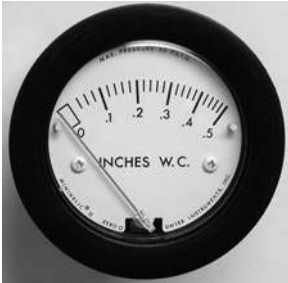
Diagram 11a: Calibration Indicator / Pressure Gauge (located below control panel at the side of the unit)
