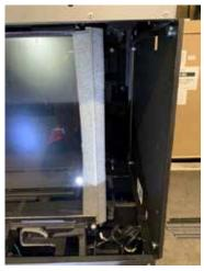
5. Screw in the three self-tapping screws at the top of the outer side panel to attach it to the firebox.
