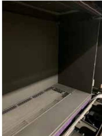
12. Once the inner side panel is wedged in place, tighten the hanger screws for the back liner panels.
