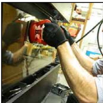
Handle glass with supplied vacuum clamps
